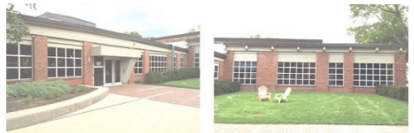
Fig. 17. We show a pair of images showing the L-shaped corner of an outdoor building, which is used in our experiment.
